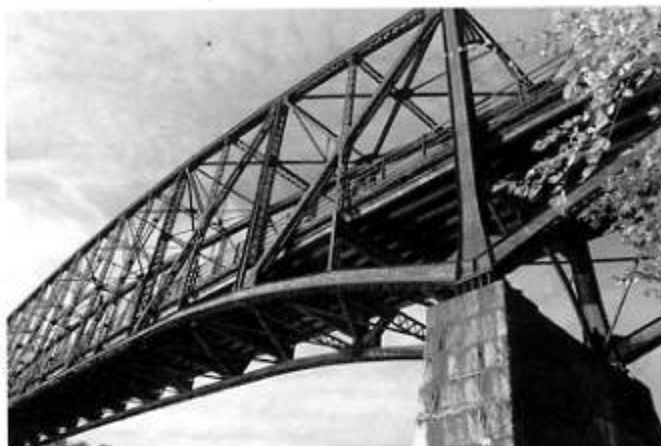
Schell Memorial Bridge, ca. 2006
