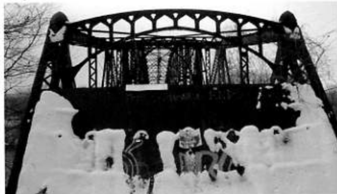
Portal of the Schell Bridge. The steel plates were welded to the bridge portals in 1987 but some of the Gothic Revival-details can still be seen.
